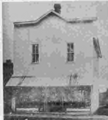
Business house in Defiance moved to Sheridan for first business house there.
