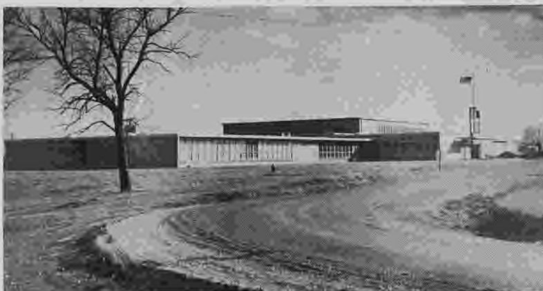
Junior and Senior High School building Worth County R-1 at Grant City.
