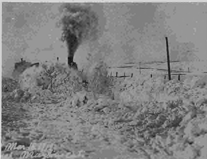
Railroad snow plow opening Maylan cut in 1912, north of Irena, Florea farm.
