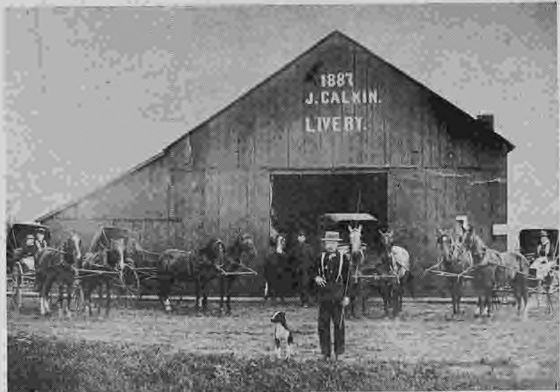
Jim Calkin's livery barn built at the beginning of Sheridan. It was by the railroad track on the old road into Sheridan from the east. At this time there was no road in front of the barn, open pasture land.
