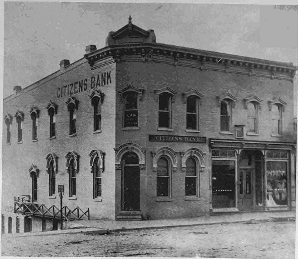
Three store buildings built by John C. Dawson, president of Citizens Bank and J. B. Dawson of Dawson's Store in 1882. After the south side fire again in 1907, J. B. Dawson and sons, Ben and C. K., housed three departments in the three buildings. This shows W. J. Gibson Law Office upstairs and Times Printing Office in basement. Note gas street light.
