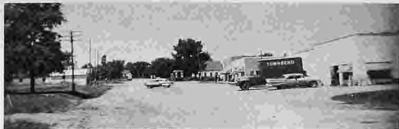
Main street of Worth rebuilt.
